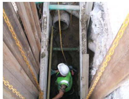
Shane Mortimer installing the new drainage
