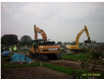
Works underway on the earthworks at the site
