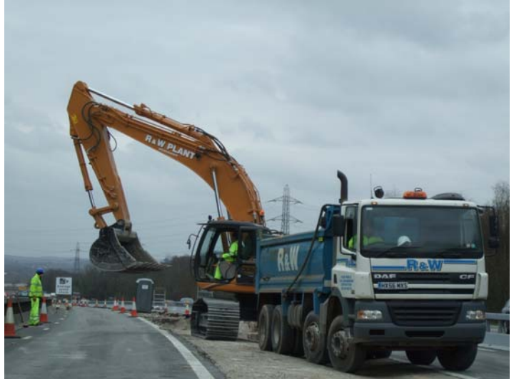
Michael Garmson, operating our new CX350, on the M27
